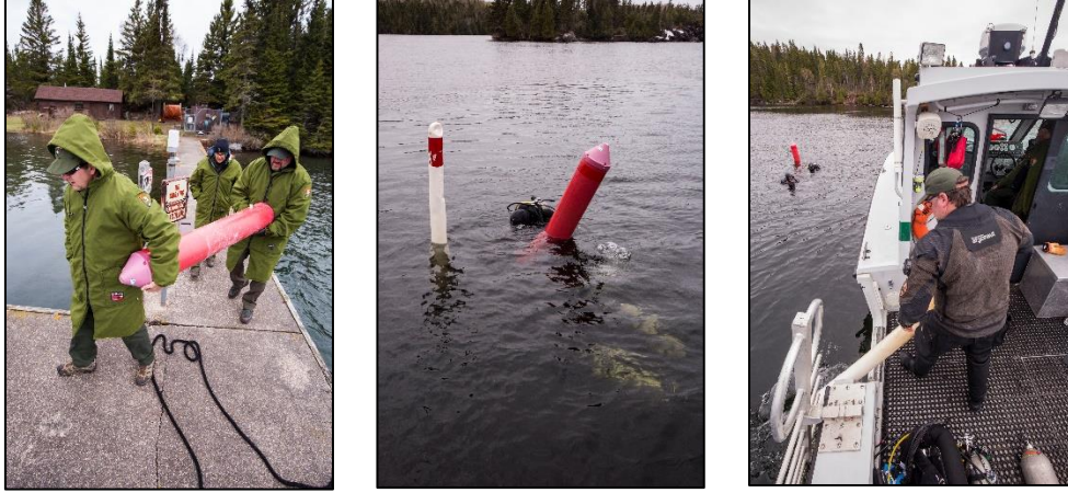
Replacement of a channel buoy
